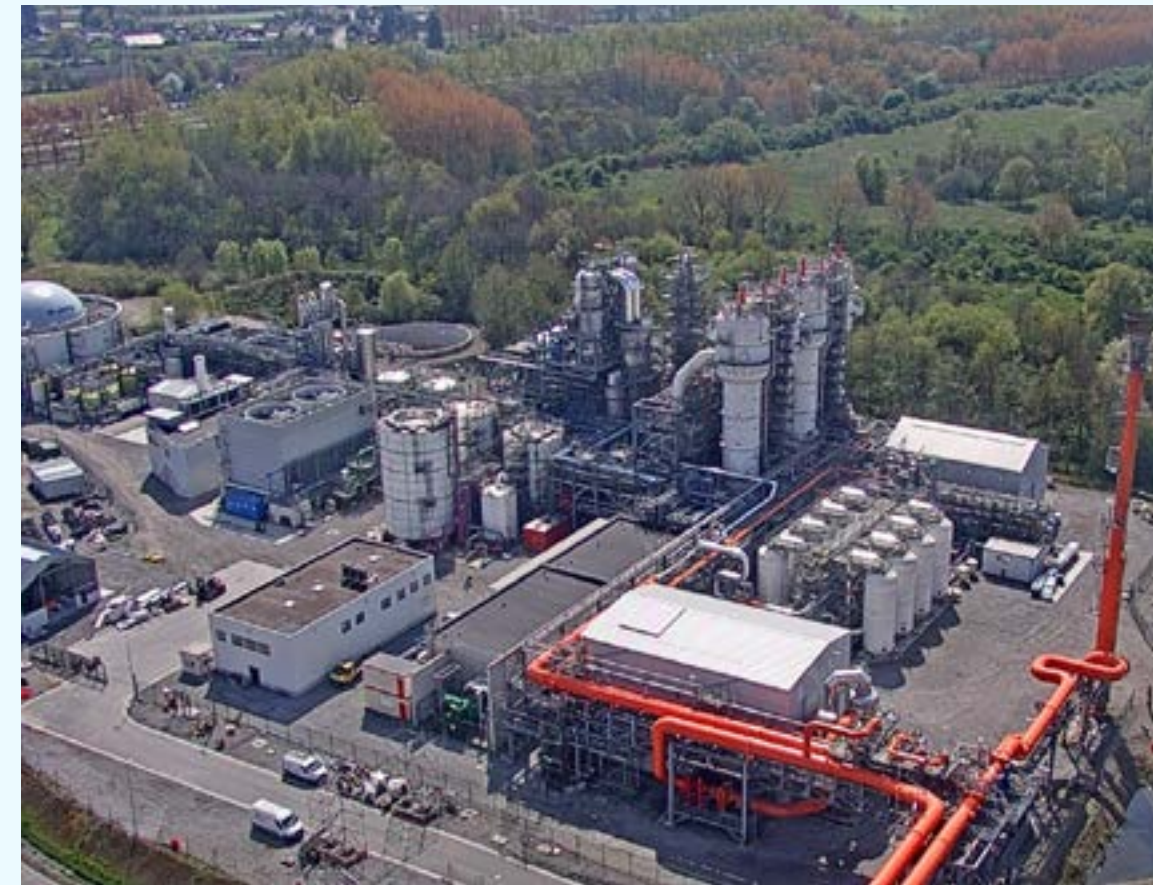
➤ The Steelanol Facility in Ghent, Belgium
