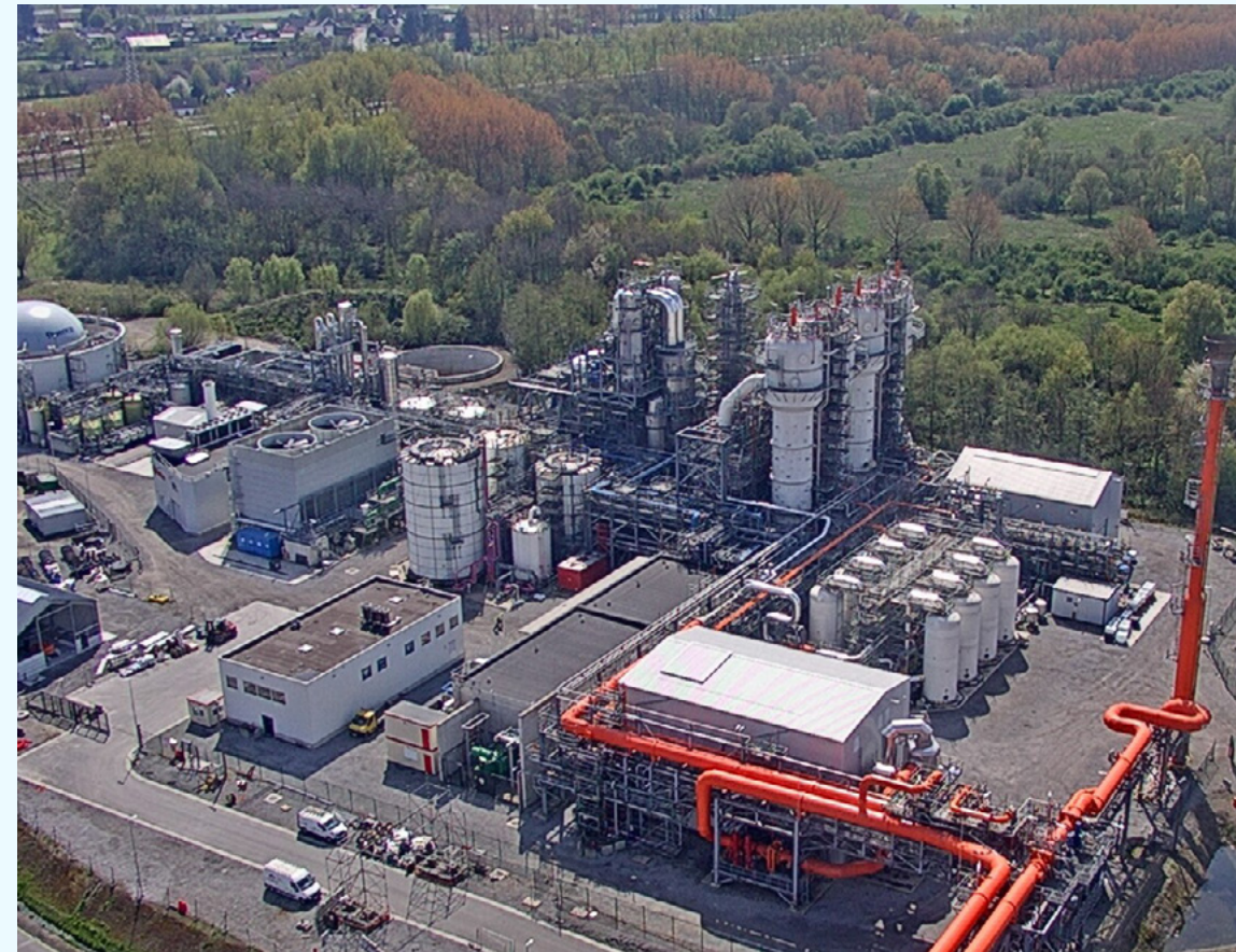
➤ The Steelanol Facility in Ghent, Belgium
